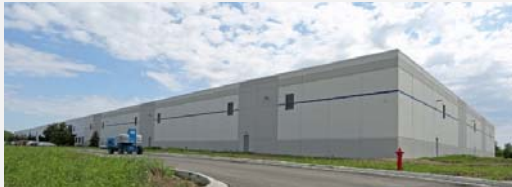
GOODWIL INDUSTRIES EXPANSION Sturtevant 115,848 SF Delivery Q4 2017
